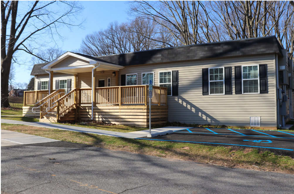
Exterior shot of the newly constructed Bear Den.
